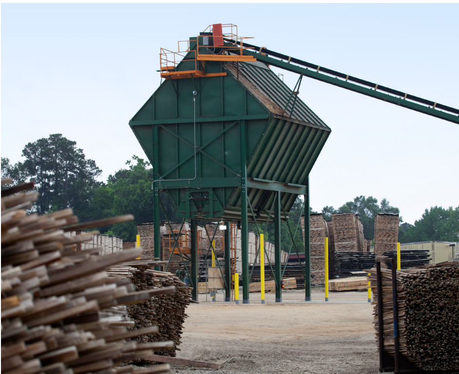
A large chip bin where all the chips from manufacturing the lumber are stored.
