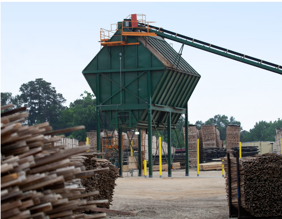
A large chip bin where all the chips from manufacturing the lumber are stored.
